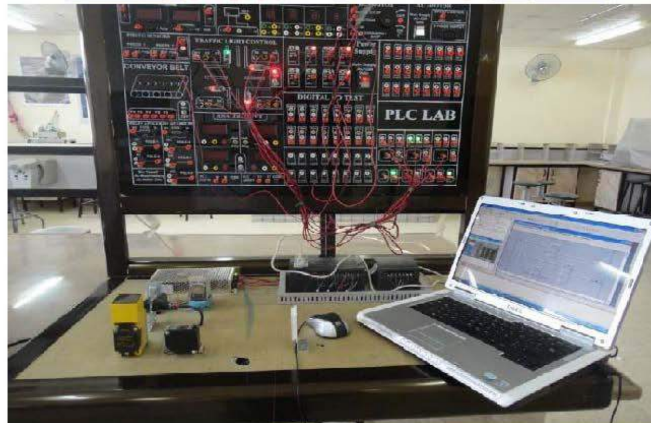
Figure 6. An Industrial PLC
